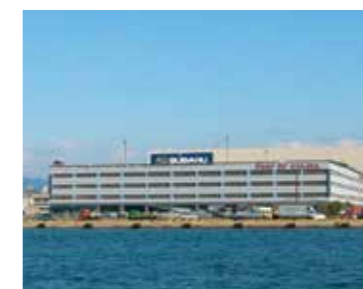
■立体車両野積場 Multistorey automobile storage facility
