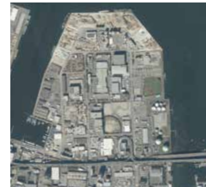
■係留施設 Mooring Facility
